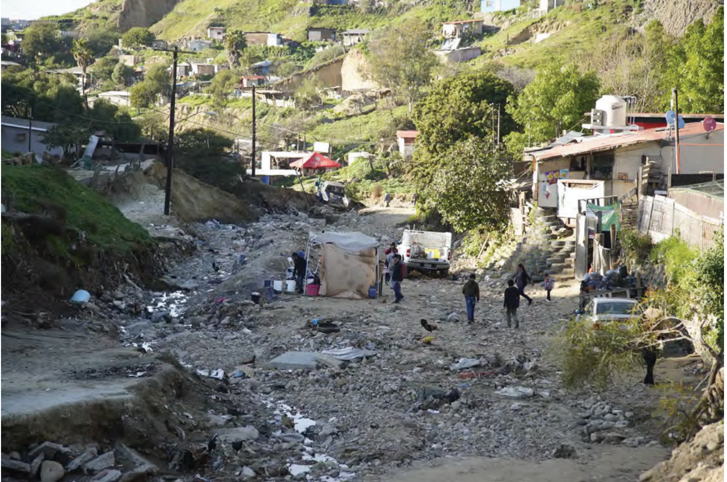
Recent rains washed over the main road leading to the migrant shelter at Templo Embajadores de Jesús, destroying water pipes and cutting off vehicle access to the shelter. (Alejandro Tamayo/The San Diego Union-Tribune)
